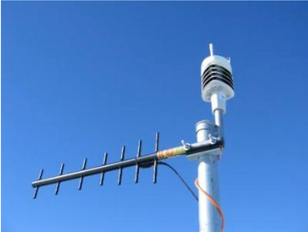
Example 2 - Vaisala welded to a pipe secured into the ground.
