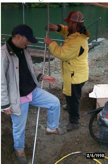
9. Repeat this process for the other 2 legs and insure they are spaced at 120 degrees off the north leg.
