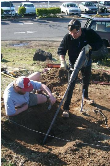
11. Use the vacuum to make sure all dust is removed from the hole and cover the holes with cardboard to make sure no rocks fall in.
