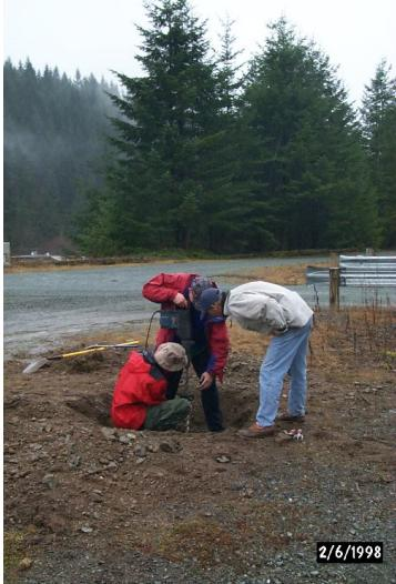
5. Temporarily set vertical steel pole in center hole, level it and keep it plumb with rags or pieces of cardboard.
