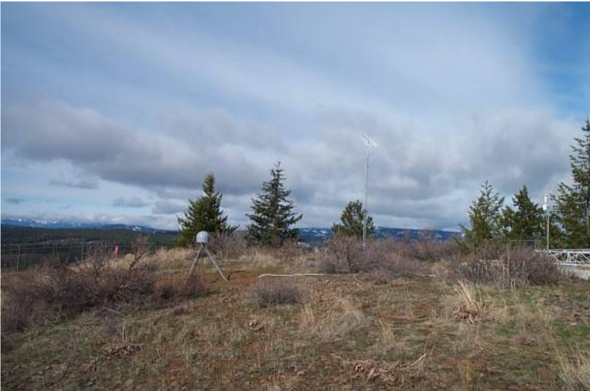
GPS station SC00 looking East. Note antenna mast for microwave link to the right of the GPS Antenna. The MET pack is at the far right of the photo.
