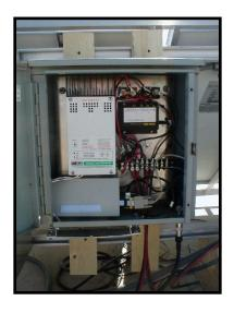
Panel: This is the power panel for the wind system. It contains a C40 Diversion Charge Controller (white w/fins), 2 shunts (black, top) to measure current from generator and solar regulator), data logger (black box, middle), 50A breaker (grey, next to C40), stop switch, Freewave radio modem (grey, bottom) and diversion load (silver, attached to bottom of box).
