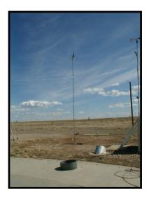
**Tower:** The tower is 24 feet tall, guyed with 4 5/32 braided stainless cable. For this setup, the anchor points are 4 30" steel auger style ground anchors. Each guy wire is approximately 21' in length. The pole is constructed of two 10' sections coupled together and one 4' section clamped to the top, attached to the generator. Three 8 guage wires run inside the tower to a junction box at the botom. where there is a lightning arrestor.
