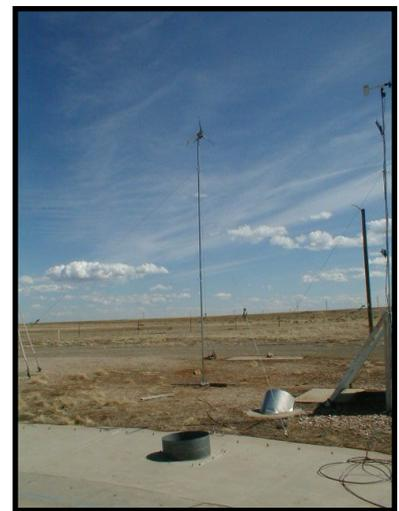
**Tower:** The tower is 24 feet tall, guyed with 4 5/32 braided stainless cable. For this setup, the anchor points are 4 30" steel auger style ground anchors. Each guy wire is approximately 21' in length. The pole is constructed of two 10' sections coupled together and one 4' section clamped to the top, attached to the generator. Three 8 gauge wires run inside the tower to a junction box at the bottom, where there is a lightning arrester.
