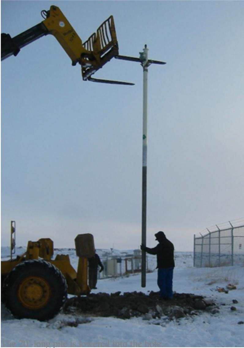
The 20'-long pile is lowered into the hole.
