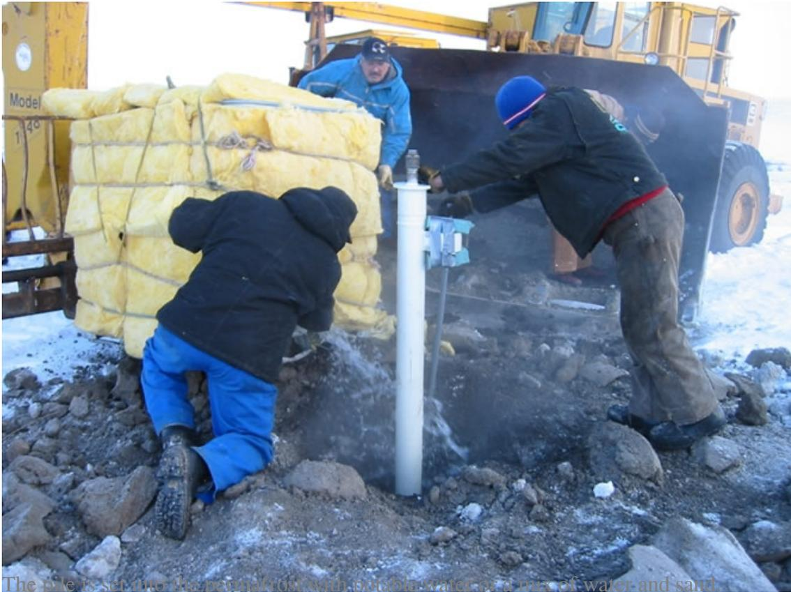
The pile is set into the permafrost with potable water or a mix of water and sand.
