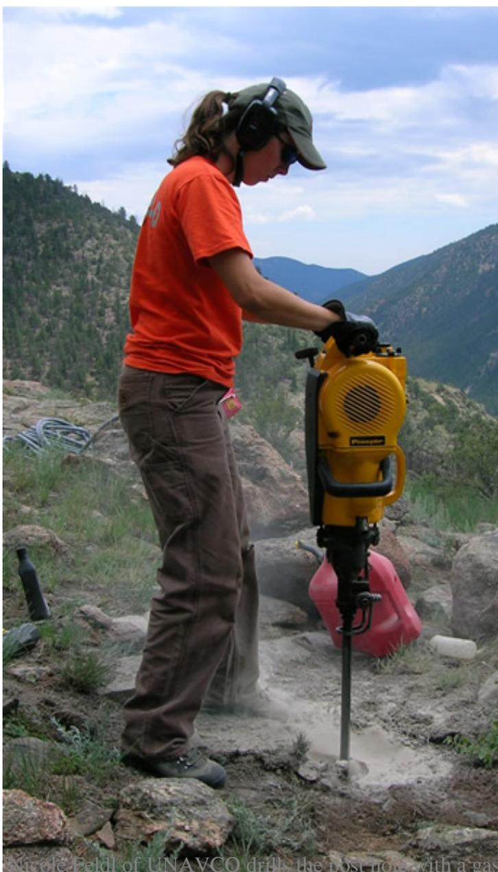
Nicole Feldt of UNAVCO drills the post hole with a gas-powered drill.
