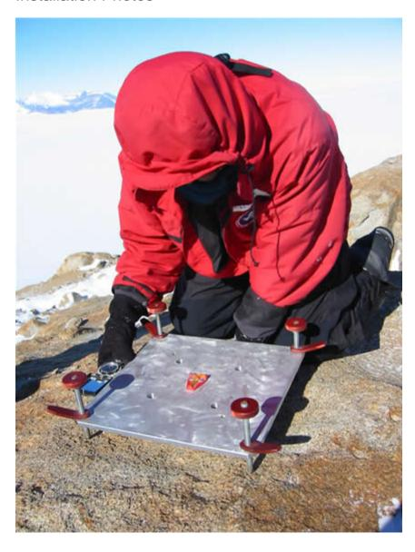
Eric Kendrick of Ohio State University works to install a mast using the custom jig on Moody Nunatak, Antarctica, as part of the WAGN network.
