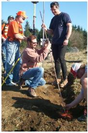
10. Remove the center leg and drill leg holes at 55 degree angle. Make sure and check the angle often with a Brunton (especially at the beginning) and have someone stand along the azimuth marks making sure the hole is in line with the center point.
