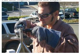
23. Place the screw thread end of the of the SCIGN adaptor (note there is a thin edge on the inside that goes up) on the center leg and tap flush.
