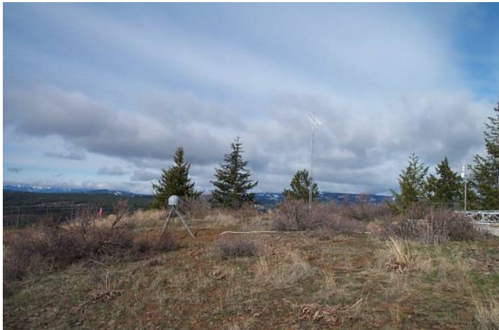
GPS station SC00 looking East. Note antenna mast for microwave link to the right of the GPS Antenna. The MET pack is at the far right of the photo.
