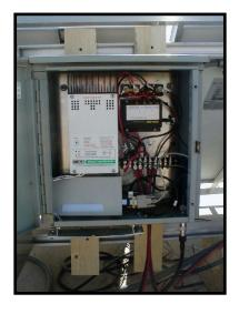
Panel: This is the power panel for the wind system. It contains a C40 Diversion Charge Controller (white w/fins), 2 shunts (black, top) to measure current from generator and solar regulator), data logger (black box, middle), 50A breaker (grey, next to C40), stop switch, Freewave radio modem (grey, bottom) and diversion load (silver, attached to bottom of box).
