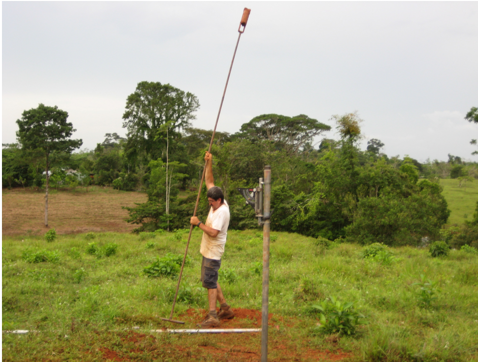
Figure 2 – Releasing the excess soli from the auger bit by pounding the handle against the ground. For this particular monument, each hole was taken to a depth of 15 feet.
