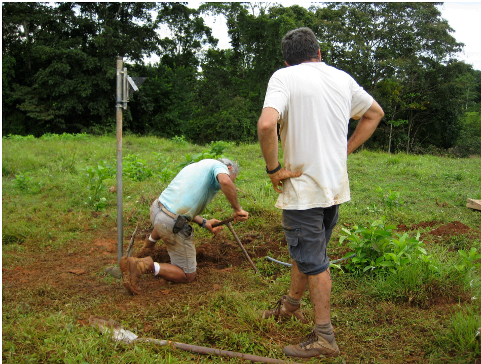
Figure 1 – Augering an angled hole for the monument. The laser beam is kept in the center of the handle for proper alignment of the hole.
